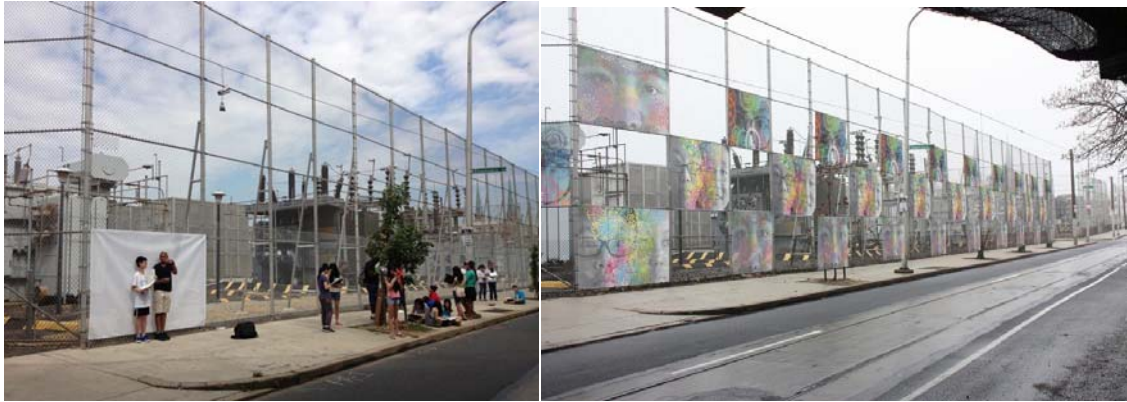
Sneak peak of the PECO Substation, before and after!
